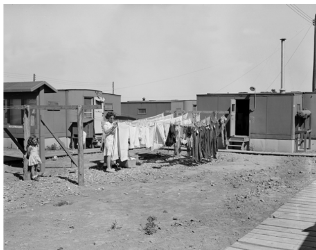
This photograph shows the type of housing that was initially constructed for the scientists and their families at Site Y.
