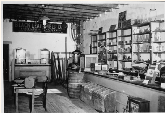
Interior of the Tunstall Store. Courtesy of Palace of the Governors Photo Archives (NMHM/DCA), No. 089736
